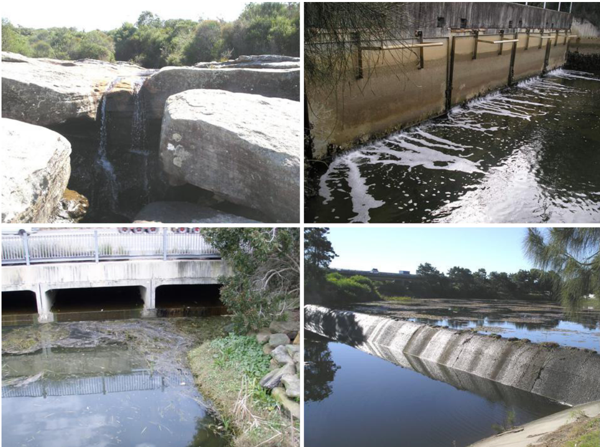
Figure 2.8.3. Fish passage barriers – natural (waterfall), floodgate, road culvert and weir.
