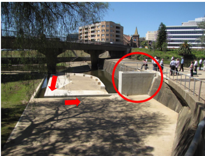
Figure 2.8.12. A fish lock fishway has been constructed at Marsden Street Weir in Parramatta. Arrows shows the entrance channel (downstream), with the lock chamber circled.
