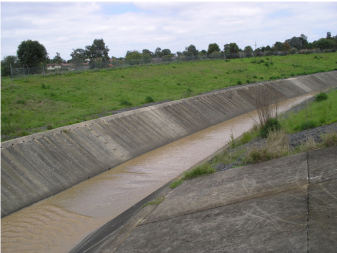
Figure 2.8.2. Bunbury Curran Creek is one of many waterways that have been channelised in the Sydney region.
