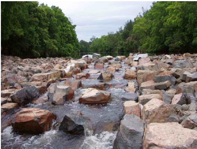
Figure 2.8.11. Full width rock ramp fishway at weir on Karuah River, Hunter region.
