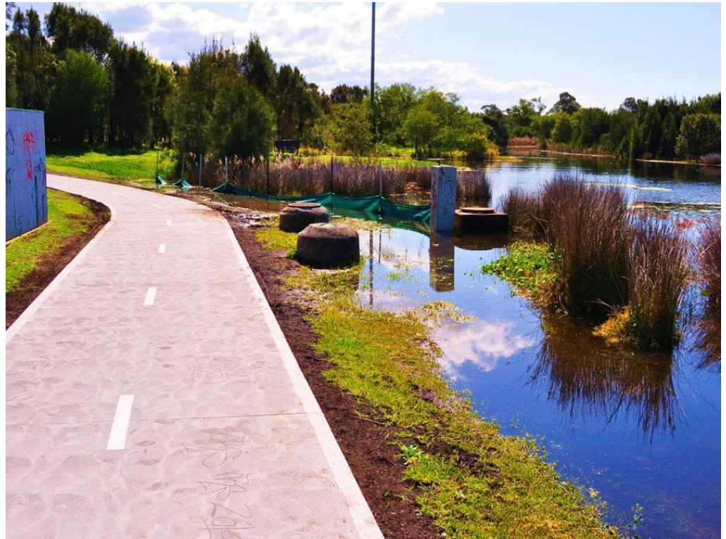
Figure 2.11.12. A combination of high rainfall and spring high tides provide an indication of the likely impact that increased rainfall intensities and projected Sea Level Rise may have on coastal wetland systems. Note the increased potential for inundation of the sewerage infrastructure, adjoining shared pedestrian cycleway and property boundaries as well as the flooding of the littoral vegetation.
