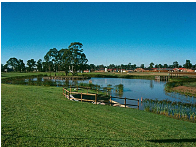
Figure 2.11.1. Plumpton Park wetlands were monitored pre and post construction. The results have been used in the development of Pollution Retention Curves by the NSW EPA and the CRC-CH. Matching aesthetic and water quality objectives requires careful design, construction and the implementation of appropriate management strategies.
