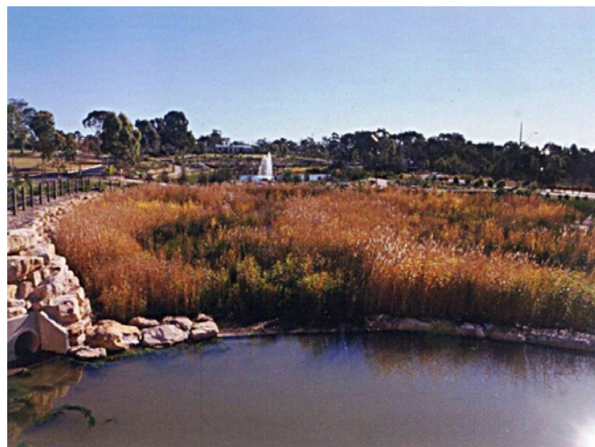
Figure 2.11.2. The WTS at Voyager Point incorporates a sediment sump, a sub-surface marsh and open water with a fountain. This system polishes stormwater from a residential catchment (approx. 25 ha) before discharging it to a highly valued and sensitive wetland (SEPP 14) downstream on the Georges River.
